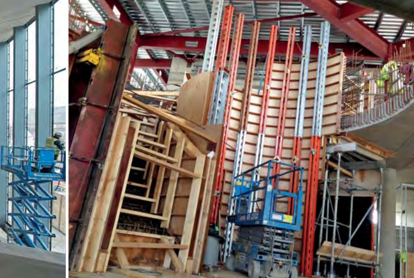
Above and left: Formwork to stairs. (Photos: BAM Construction.)
